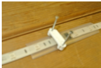
secure strip with nailing clip
